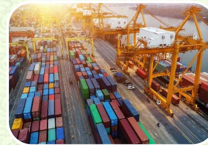
Construction of Seaport, River Port and Dry Port
