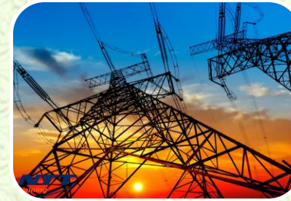
Power Generation, Transmission and Distribution
