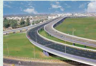
Construction of Road, Bridge and Railway Line
