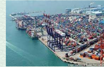
Construction of Seaport, River Port and Dry Port
